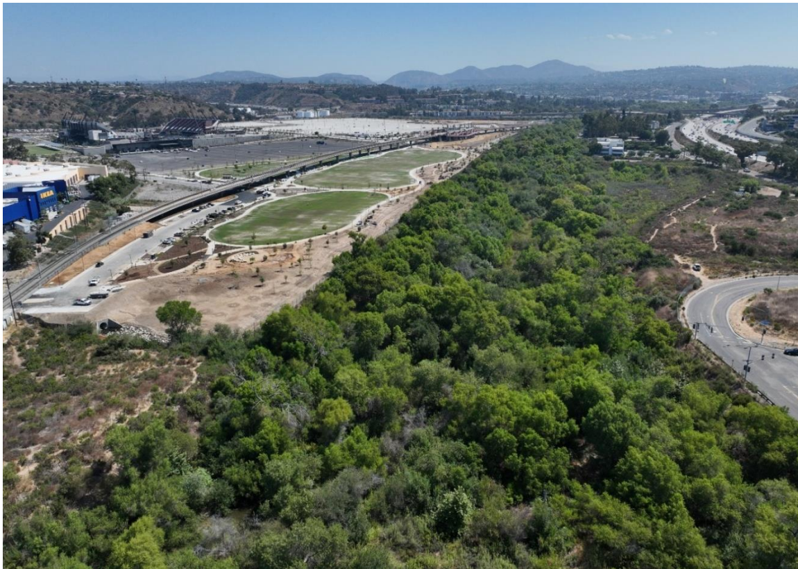
Fenton Parkway Bridge location and San Diego River.
